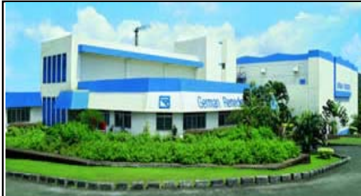
Finished Dosage Form, Goa
